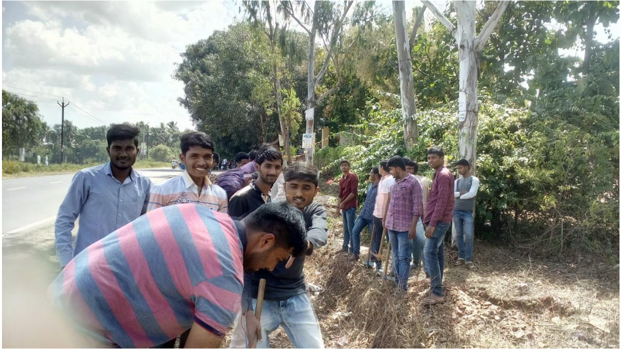
Pic 03 : Cleaning at outside main gate area
